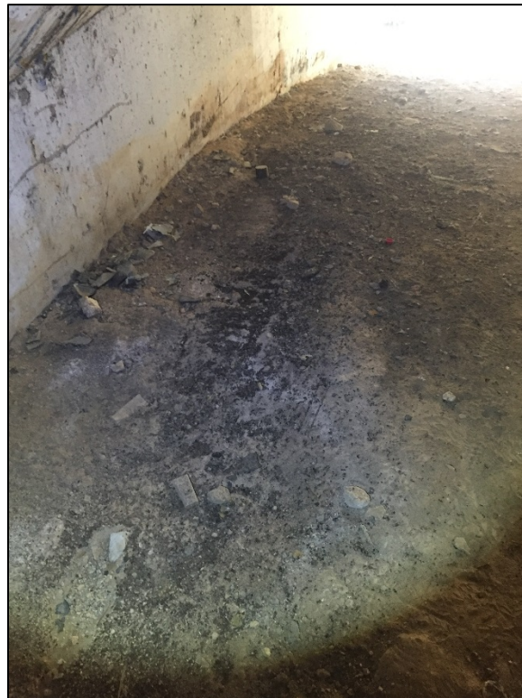
Figure 6. Guano accumulation beneath Oak Grove Drive bridge
